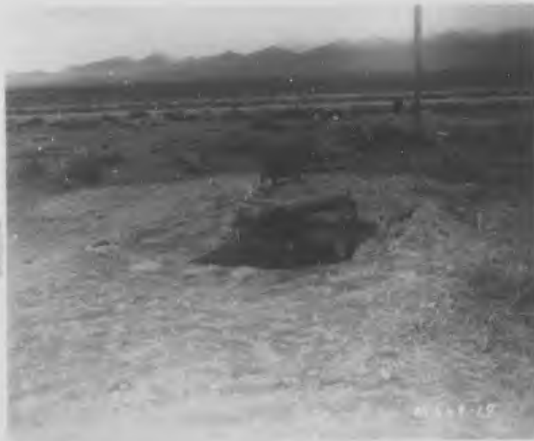
Before ↑ Heavy Machine Gun Emplacement After ↓
